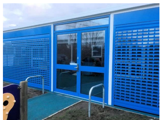
Figure 3: A close up of the commercial fire doors and secure roller shutters on the canopy
