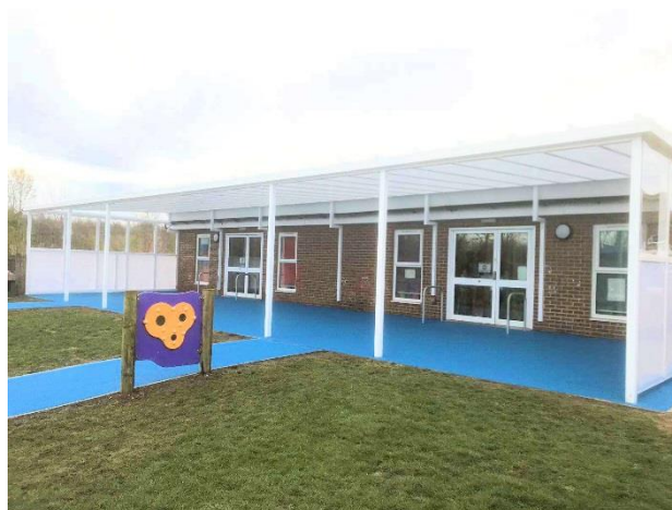
Figure 1: The new canopy with soft play safety surfacing
